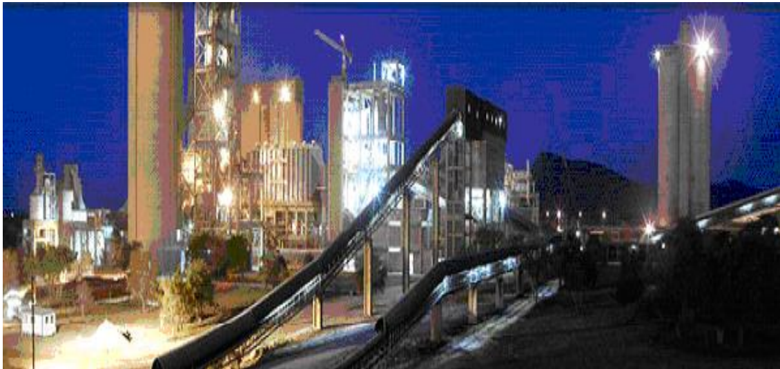
Fig. 4.8 A cement manufacturing plant
